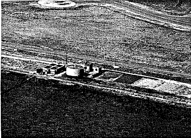
HAMILTON AIR FORCE BASE sewage treatment plant discharges effluent to the shallow waters of San Pablo Bay after primary treatment. Secondary treatment will soon be added.
