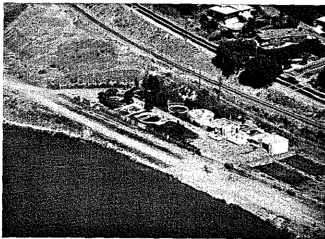
TRESTLE GLEN PLANT of Richardson Bay Sanitary District provides secondary treatment for a dry weather flow of 0.15 mgd.
