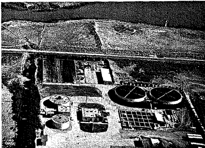
MILL VALLEY SEWAGE TREATMENT PLANT provides secondary treatment for sewage from communities at the head of Richardson Bay.
