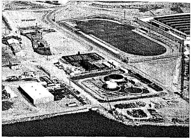
SAN QUENTIN PRISON sewage treatment plant serves the prison community. After intermediate treatment the sewage is discharged to the adjacent shallow waters of San Francisco Bay.
