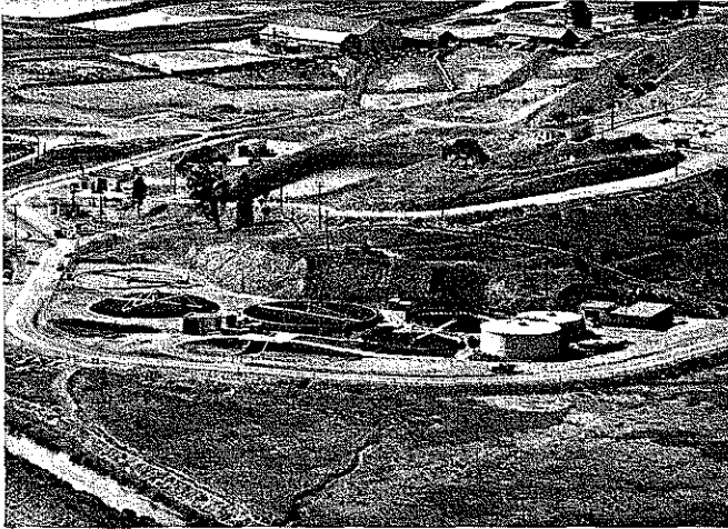
TREATMENT PLANT of the Las Gallinas Valley Sanitation District employs the biologic filtration process for secondary treatment and discharges to the shallow waters of San Pablo Bay.
