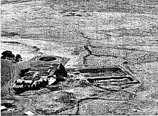
TWO TREATMENT PLANTS of Sanitary District No. 6 discharge effluent to Novato Creek. The Novato plant (left) has a design capacity of 2.7 mgd, and the Ignacio plant (right) is designed for 0.9 mgd. Both plants provide secondary treatment.
