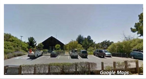
SBCWD Administrative Offices
